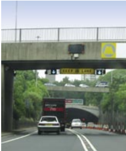
Entrance to Kingsway Tunnel
